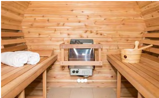
Inlet under electric heater on Back wall
